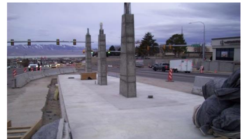
Provo-Orem BRT Platform Construction
